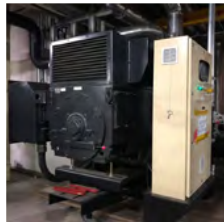
Purchased a new 500hp air compressor to replace three 200hp compressors
